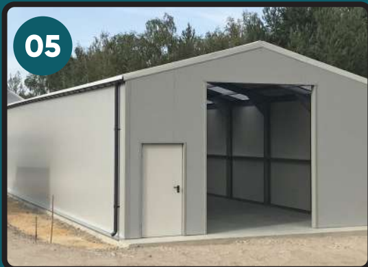
Insulated Storage Building
